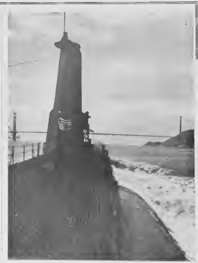
LARGE BELLY: The U.S. Navy's new underwater tanker, USS Guavina served aboard in sight of the San Francisco Bridge. The craft, built and proved admirably during World War II, was converted in 1943. Large saddle tanks have been hung on her sides and smaller tanks placed inside her hull to carry fuel.
